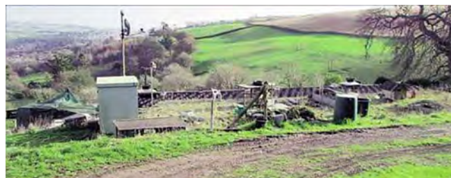
Top of the reservoir
